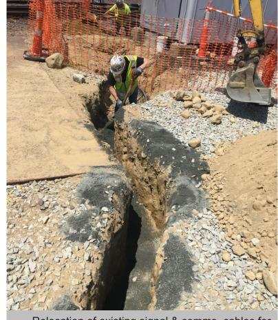
Relocation of existing signal & comms. cables for new CBH and CIH
