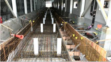
Track 11 Building Expansion – Rebar and concrete placements for inspection pit, slab, and walls
