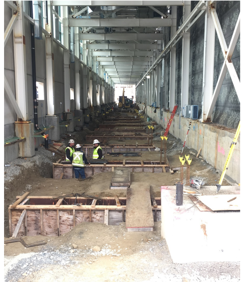
Building Expansion Pile Caps for Track Beam
