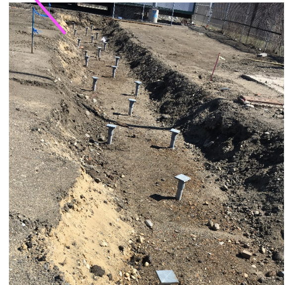
Helical Piles Completed at Parts & Storage Building
