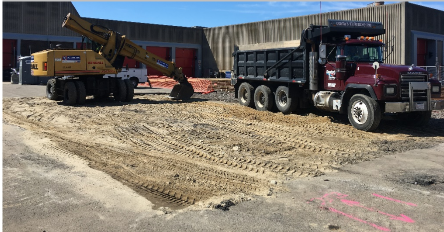
Demolition for Substation, Generator, and Ductwork
