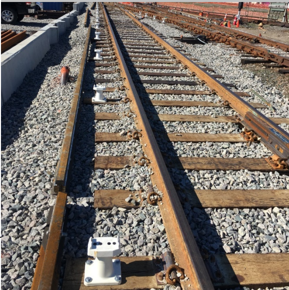
Loading Track - Starting to lay insulators & third rail
