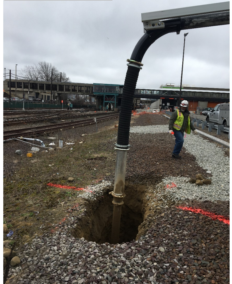
Performing Test Pits
