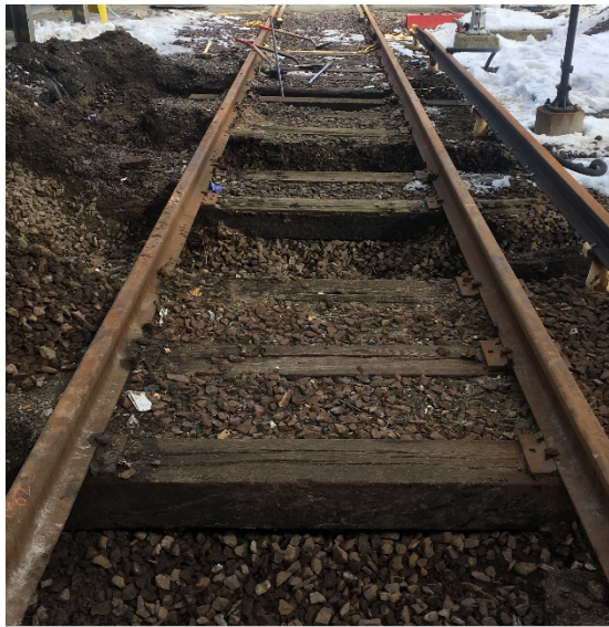
Track 13 Tie Replacement
