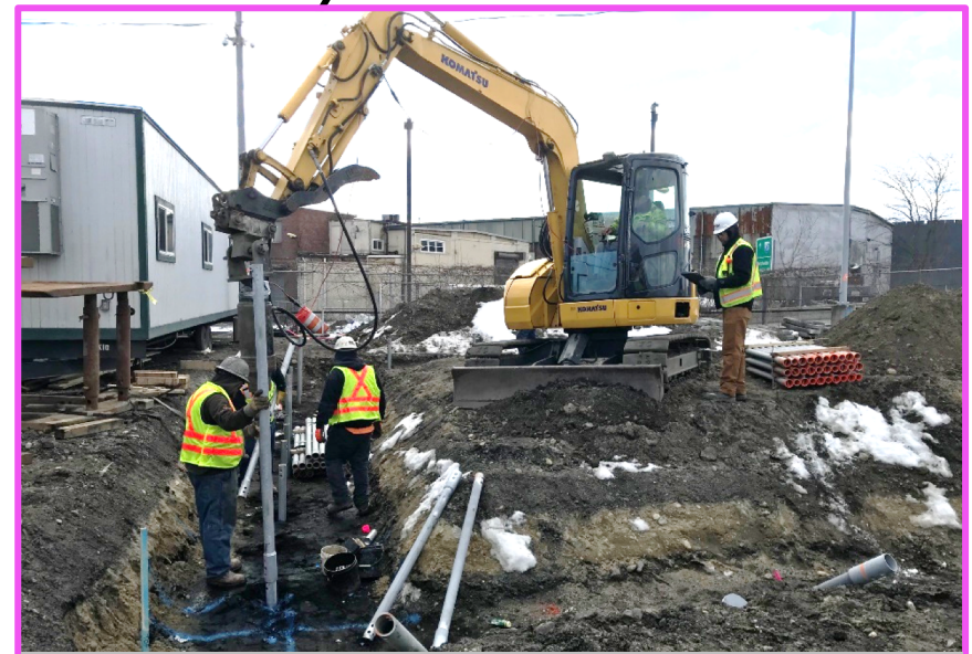
Helical Pile Installation at Parts & Storage Building
