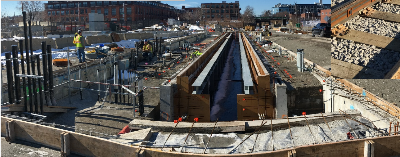
Yard 61_VTF_Plumbing & Flow Fill
