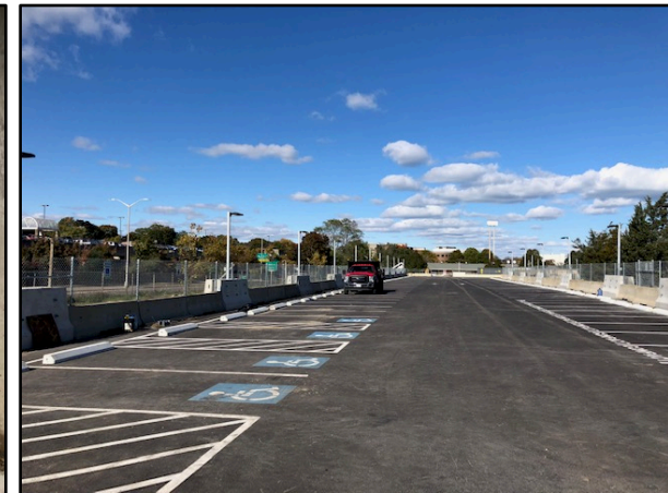
New Parking Lot at Ivory St
