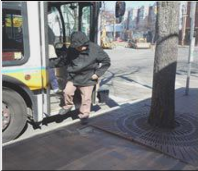
Tree Grate Tripping Hazard
