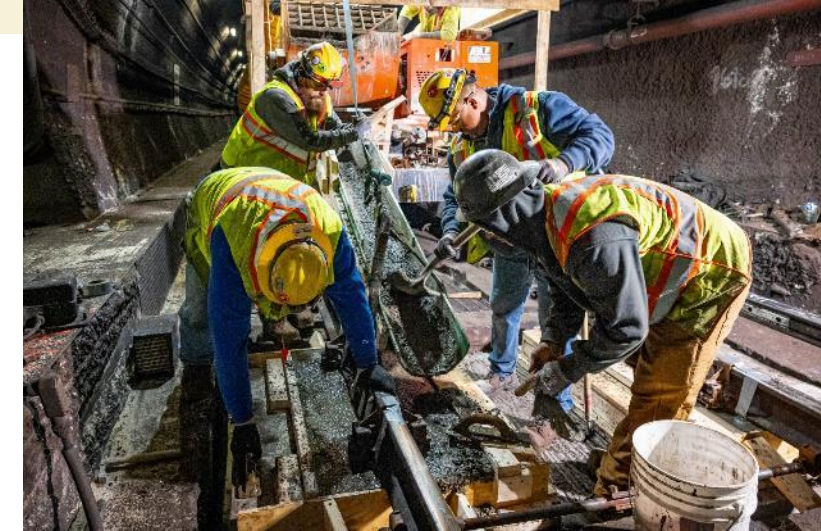
Repairing concrete slabs
