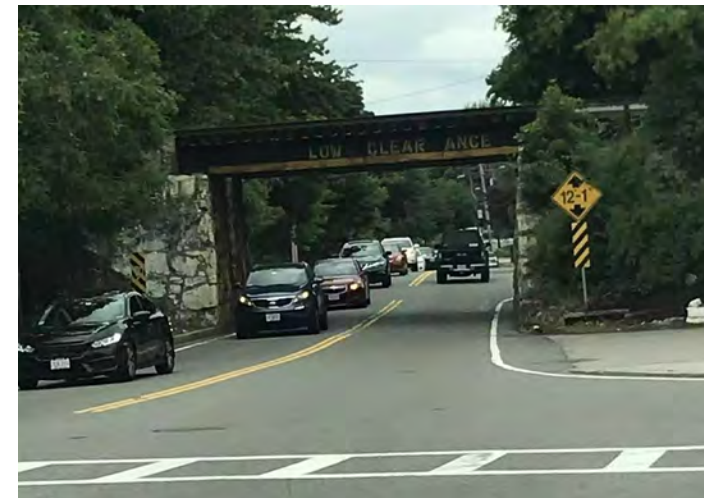
Looking west on East St.
