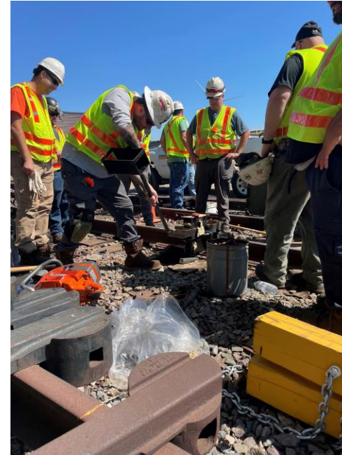
Thermite Welding
