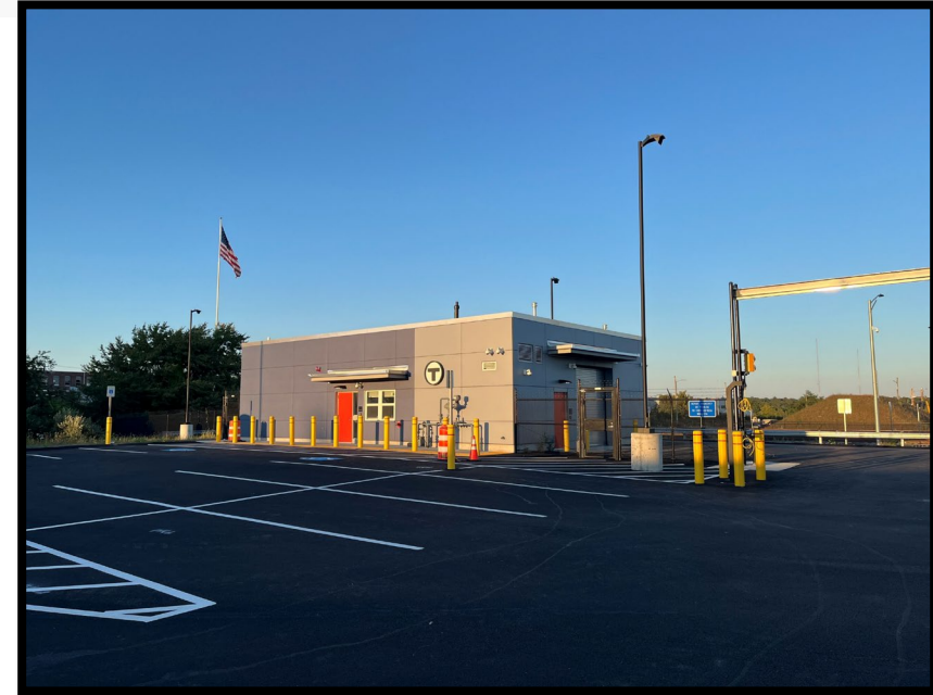
Crew building at Wamsutta Layover
