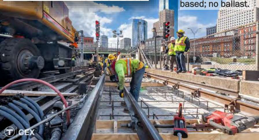
Track base in this area is concrete based; no ballast.
