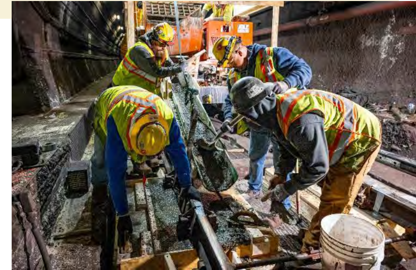
Repairing concrete slabs
