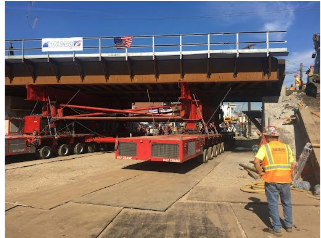
SPMT Bridge Move Example
