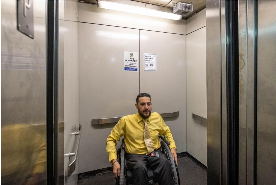
A rider who uses a wheelchair mobility device in an MBTA elevator with a urine detection sensor on the ceiling (top right).
