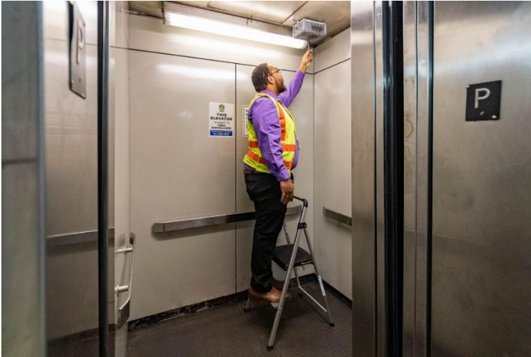
A Transit Ambassador Manager standing on a step stool in an elevator to hard reset a urine detection sensor
