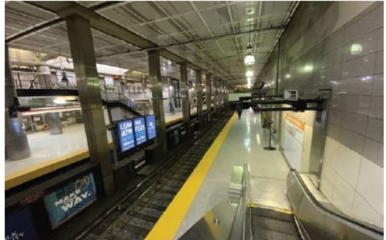
Orange line Outbound Platform and Existing Escalator
