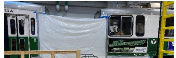
Abatement area quarantined between two vehicles
