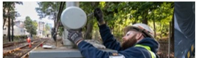
GLTPS equipment installation during D Branch surge
