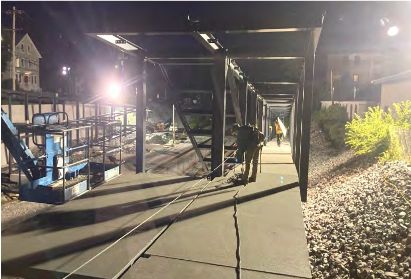
Contractor working on the inbound ramp
