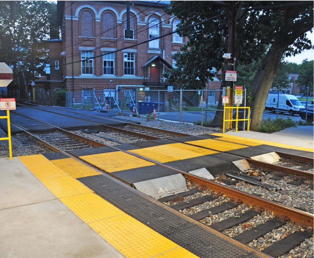
Track crossing at Brookline Hills Station on the Green Line
