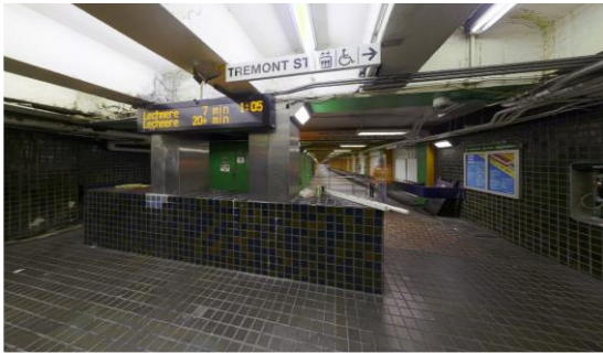
Park Street existing conditions
