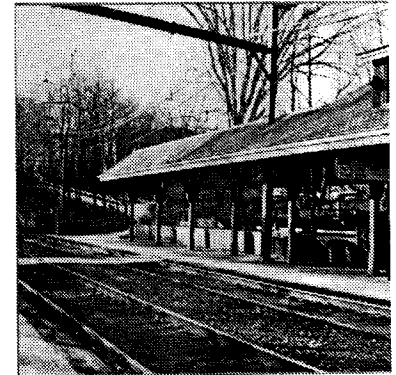
Fig. 2-115 Existing Canopy at Newton Center
