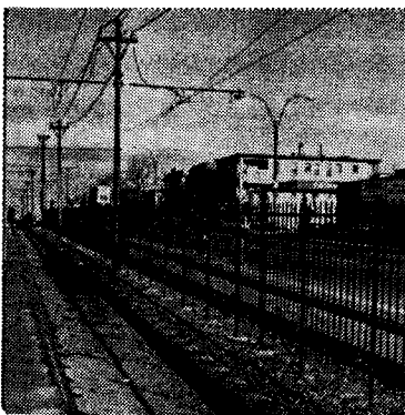
Fig. 2-136 Existing Mid-Track Fencing
