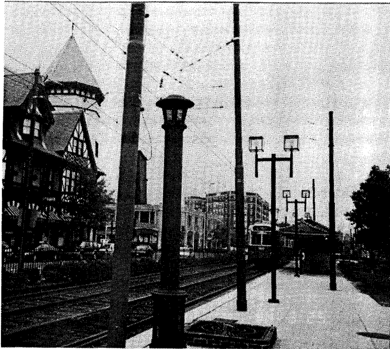
Fig. 2-112 Existing Platform Lighting Fixtures at Coolidge Corner
