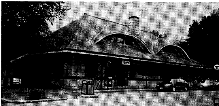
Fig. 2-117 Existing Shelter at Newton Center Station
