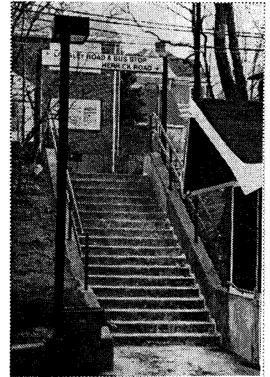
Fig. 2-53 Existing Stairs at Newton Center
