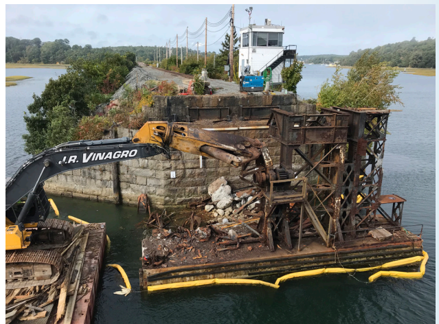
Demolition of Pier 1 trunion tower
