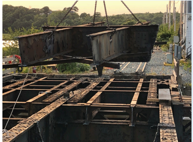
Removal of Bascule span framing
