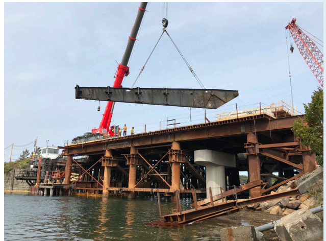
Bascule girder removal
