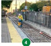
Between Melvin Avenue and Washington Street, crews performed thermite welding, grinding the welds down to provide a smooth ride for Green Line passengers [Picture | 3] and ultrasonic testing [Picture | 4]
