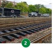
Between Summit Avenue and Washington Street, crews worked on track demolition [Picture | 1]. Rail, ties and ballast were successfully removed. The sub base was compacted and new ties were installed [Picture | 2]
