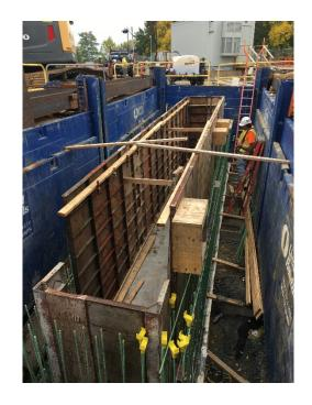
Contractor started work in Zone C (Tracks 12 – 14), working on concrete work for the Circuit Breaker House foundation in the South Yard, ductbank work being performed, and site lighting is 99% operational.
