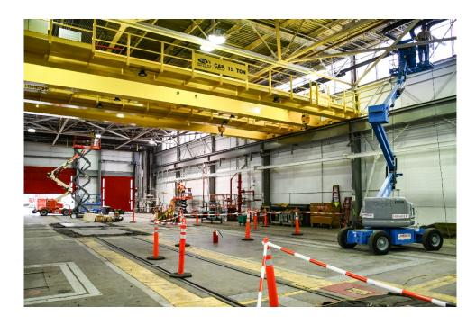
The contractor is currently working in Zones C & F of the maintenance facility and replacing track in Zone C in the yard. Two new 15-ton cranes were installed and the programming was completed for the alarm(s) and safety devices.
