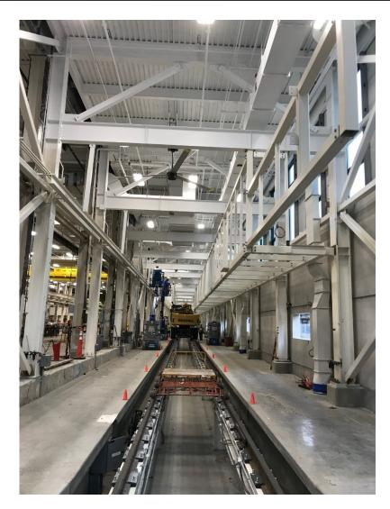
Continued work on the Track 11 bay building addition such as suspended catwalk structural steel, approach slabs, and door installation at the north end.
