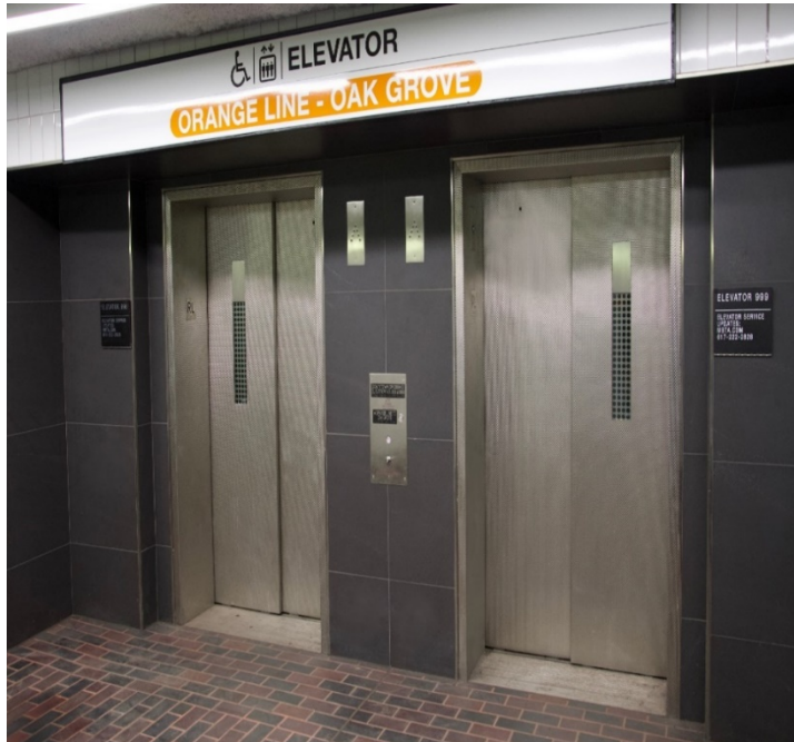
New DTX Elevator Nos. 998 and 999 at Redline Northbound Passageway
