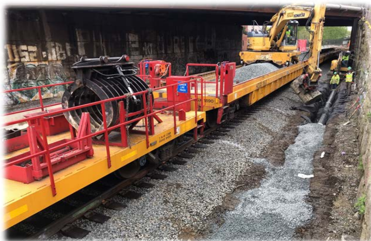
DB Entity – Medford Street – Installing Temporary Drainage
