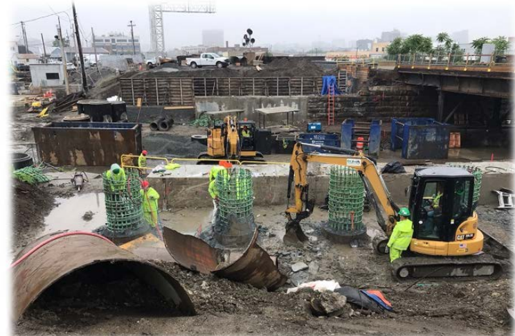
DB Entity – Washington Street Bridge – Chipping concrete, grading
