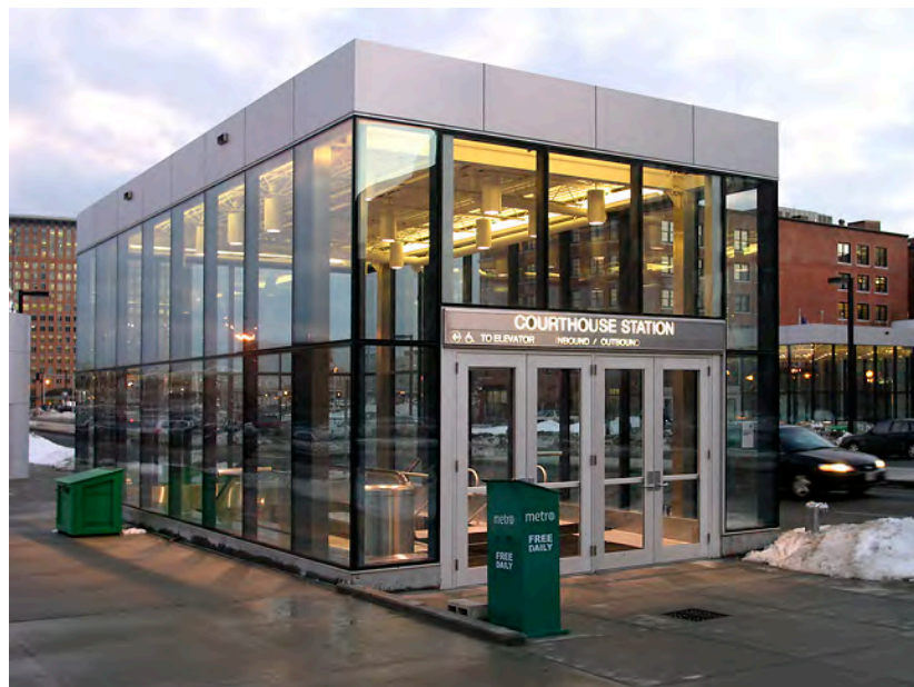
Courthouse Station (Silver Line)
